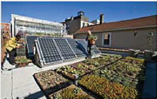
Solar panels on the roof are tilted to the heavens, and trays of artificial soil are planted with sedum and other plants to soak up rainwater and keep it from flooding the city's storm drainage system. Michelle Litvin for The New York Times
